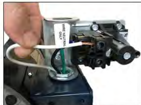
4. Remove yellow wire nut from motor NEUTRAL.
