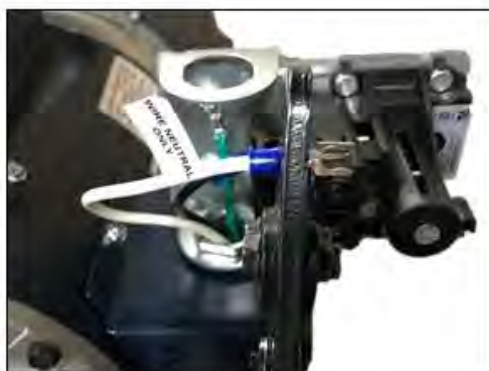
5. Crimp a spade connector onto NEUTRAL wire.
