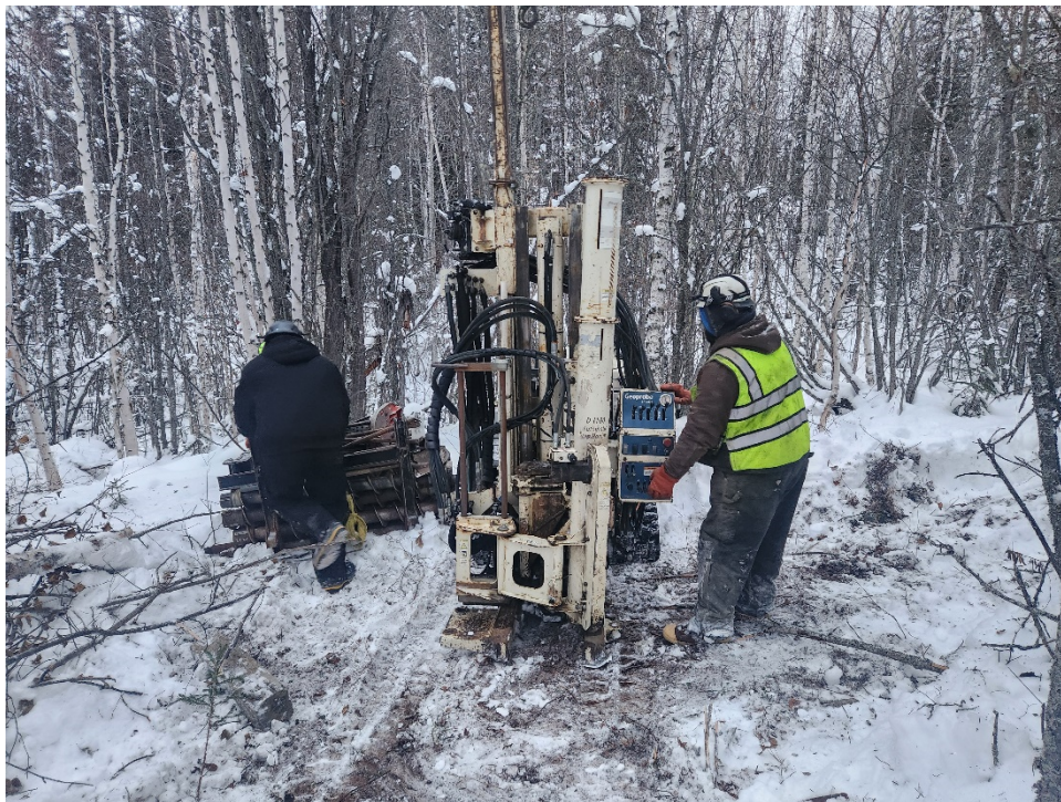
Photo C - 1. BH-01 Drill Rig Set Up
