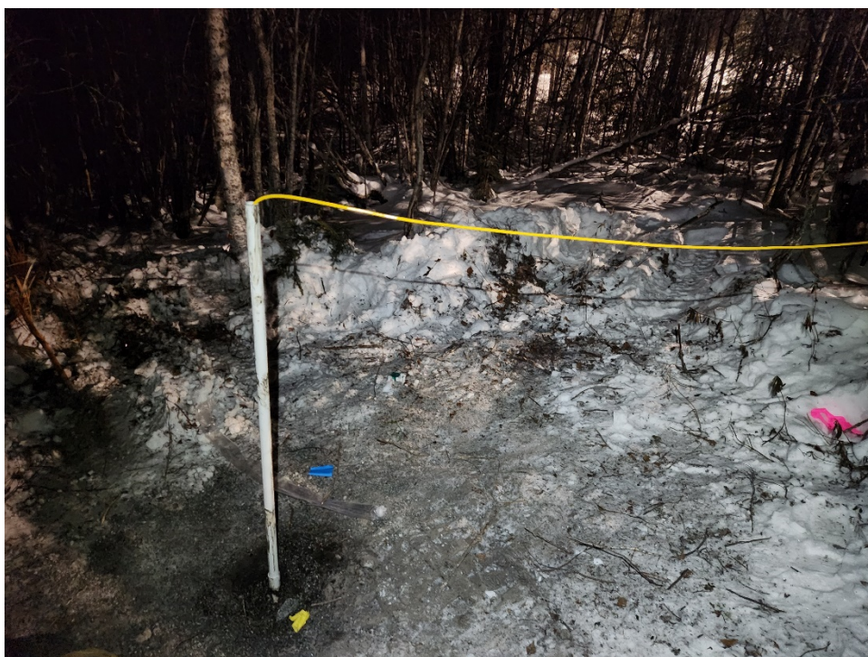
Photo C - 2. BH-01 PVC Stick Up and Thermistor String Installation
