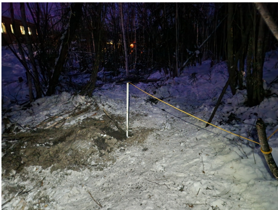
Photo C - 6. BH-03 PVC Stick Up and Thermistor String Installation
