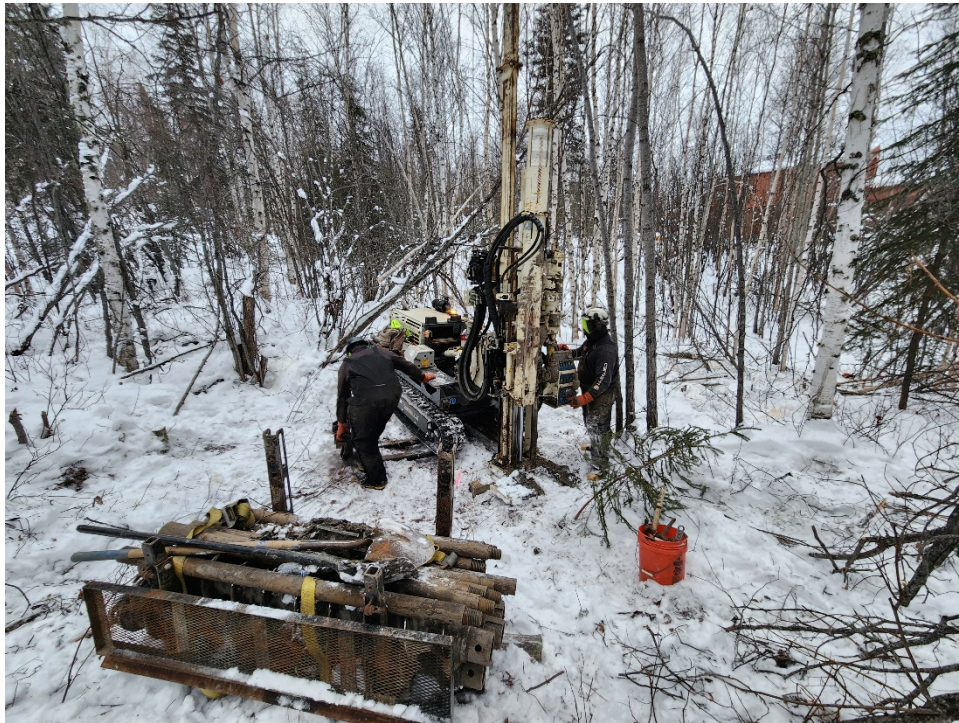
Photo C - 3. BH-02 Drill Rig Set Up
