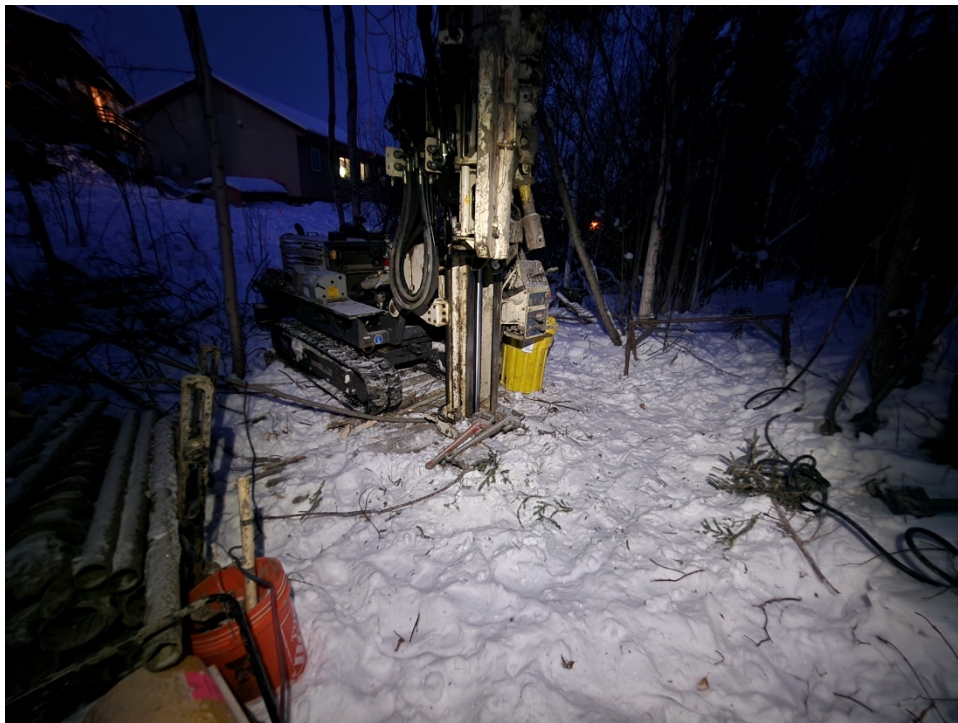
Photo C - 5. BH-03 Drill Rig Set Up
