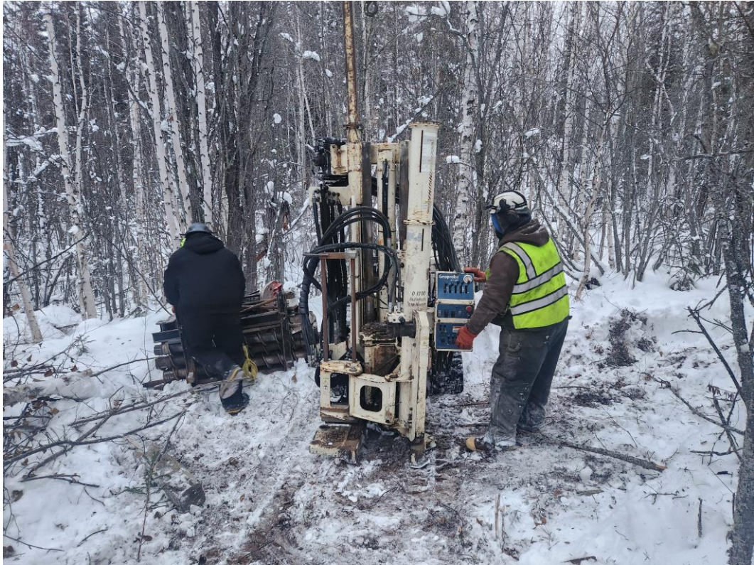
Figure 6: DD's Geoprobe 6712DT Drilling at Borehole BH-01
