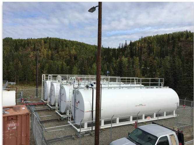
Figure 28 New 80,000-gallon Farm Tanks
