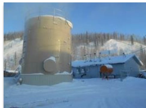
Figure 25 Water Tank 40,000-gallons.
