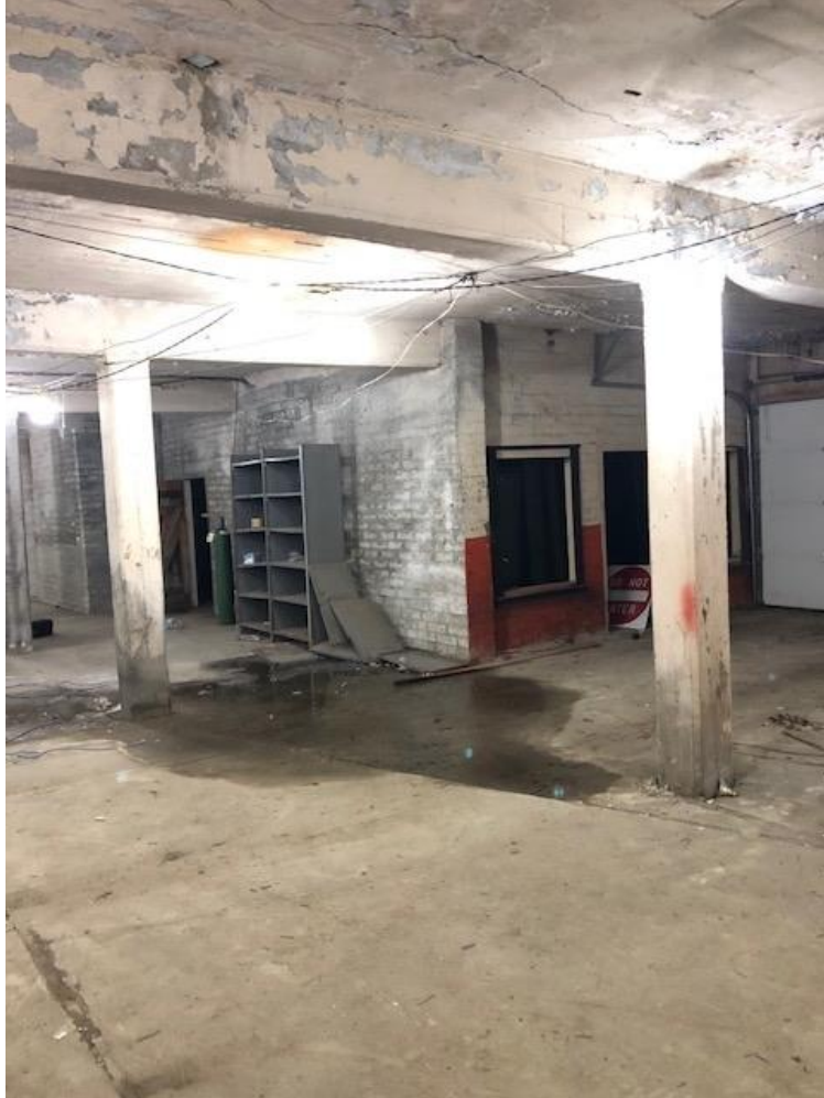
Northwest Interior View
