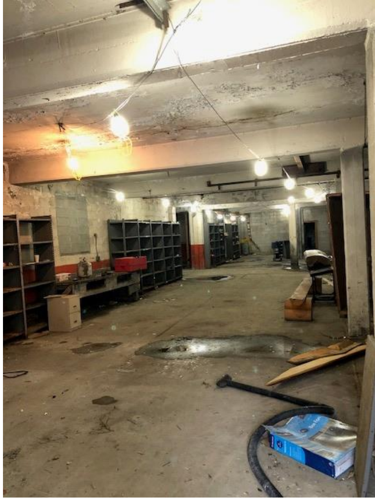
North Interior View
