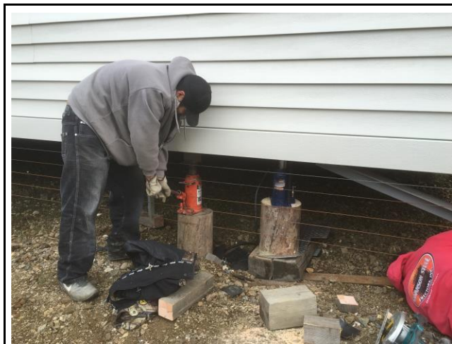
#9 Jacking arrangement
