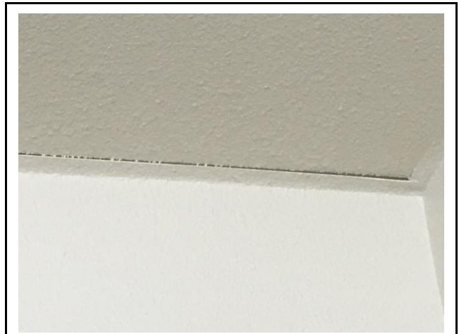
#8 Gap at wall/ceiling intersection in waiting area
