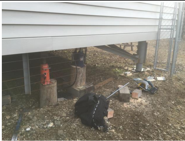
#3 Blocking sunk into gravel 4" to 6" under pressure
