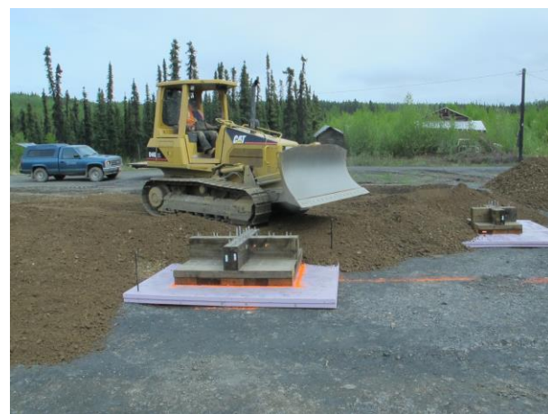
#5 Timber footing installation
