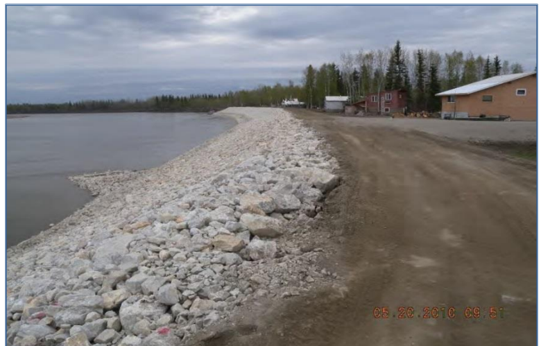
Figure 4-1 Phase 1 NCRS Riverbank Stabilization Project
