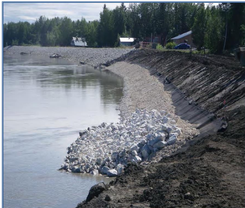
In 2015, NRCS assisted McGrath with reconstruction of a protective levee along Takotna Avenue to prevent flooding and erosion.
