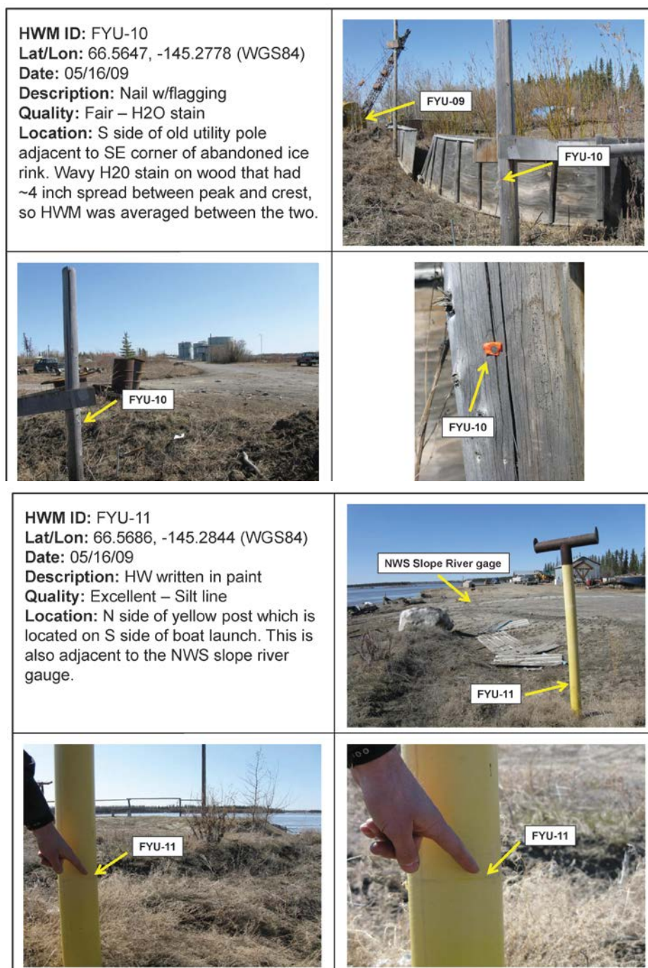
Figure 5-6 Fort Yukon Flood Impacts (NWS 2009)
