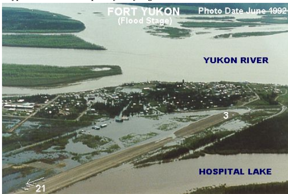
Figure 5-9 1992 Fort Yukon Flood (FAA 2010)
