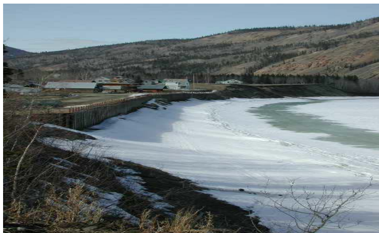
Photo 2: Sheet pile retaining wall along the city of Eagle shoreline protects the bank from erosion. The unprotected high bluff area is in the background, beyond the end of the sheet pile wall; photo courtesy of the Division of Homeland Security and Emergency Management, 2001”(USACE 2008).
