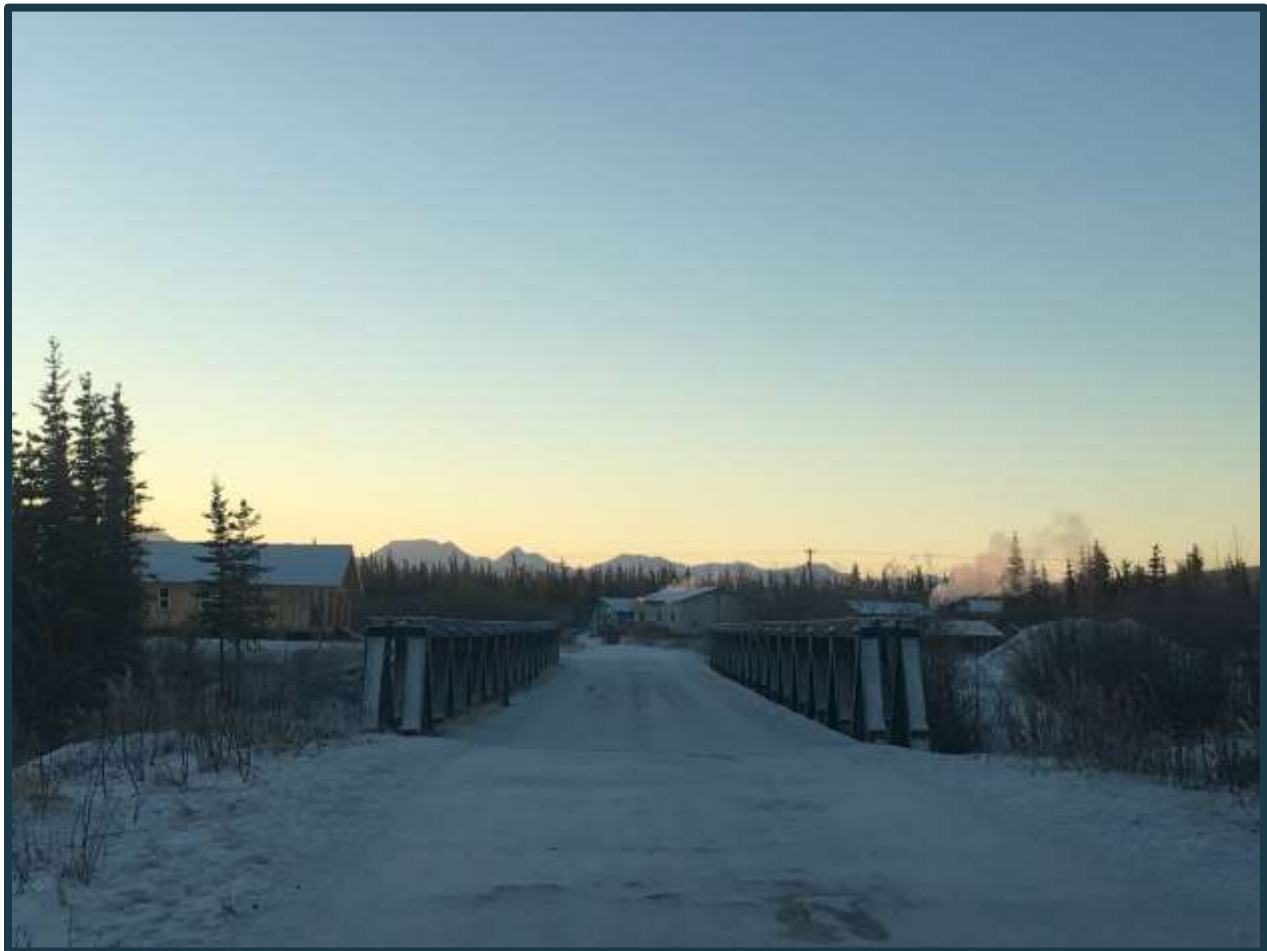
Bridge in Tetlin
