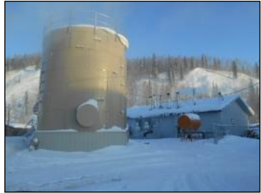
Figure 20 Water Tank 40,000-gallons
