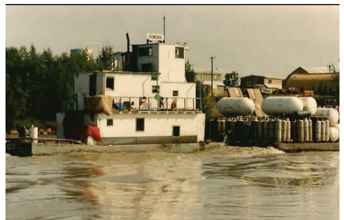
Ramona landing in Tanana. Photo Courtesy of Doug Sturm
