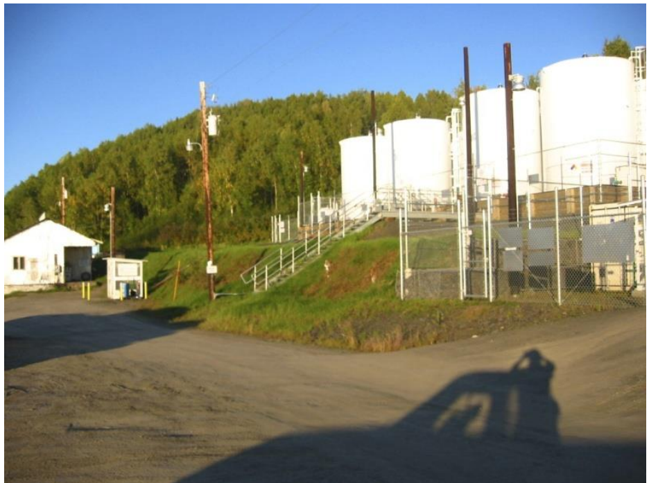
Dineega Fuel Tanks
