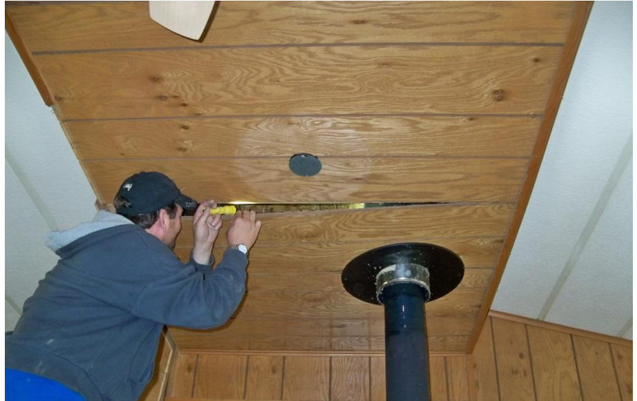
IRHA Weatherization Improvements on Ruby Home
