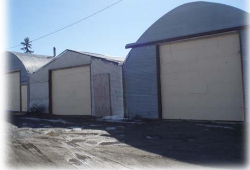
Fort Yukon Biomass Project (Ongoing)
